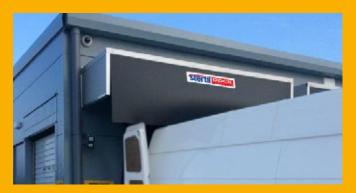
Specially designed roof to prevent against wind and rain
